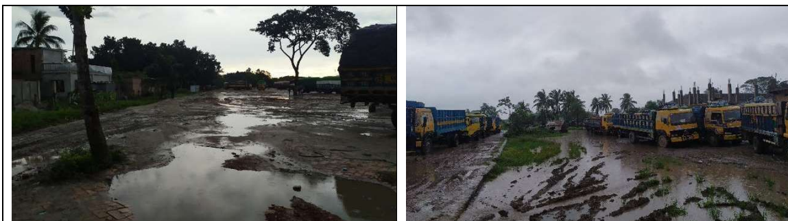
Figure 4.3: Drainage Status of the Project Areas
